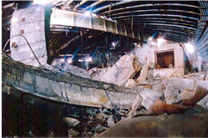
*FIG. 6.4. Reactor room of Unit 4 after the accident.*
