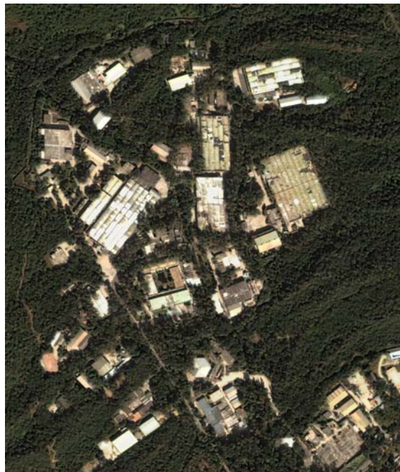
Kahuta gas enrichment facility, October 19 2005; Image credit Digital Globe-ISIS
