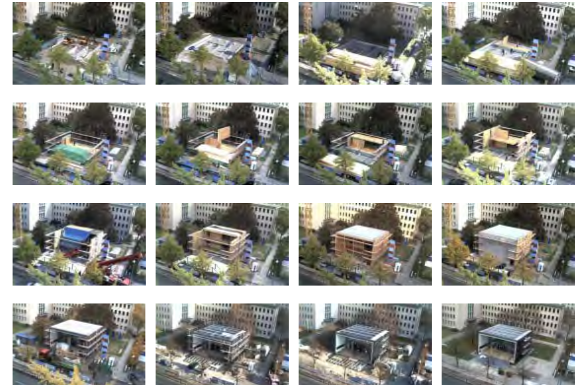
Fig. 58: Erection sequence, August, 2011, through November, 2011
