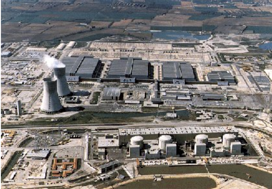
The large Georges Besse I enrichment plant at Tricastin in France (beyond cooling towers) was shut down in 2012. The four nuclear reactors in the foreground provided over 3000 MWe power for it.
