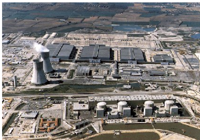
The large Georges Besse I enrichment plant at Tricastin in France (beyond cooling towers) The four nuclear reactors in the foreground provide over 3000 MWe power for it.
