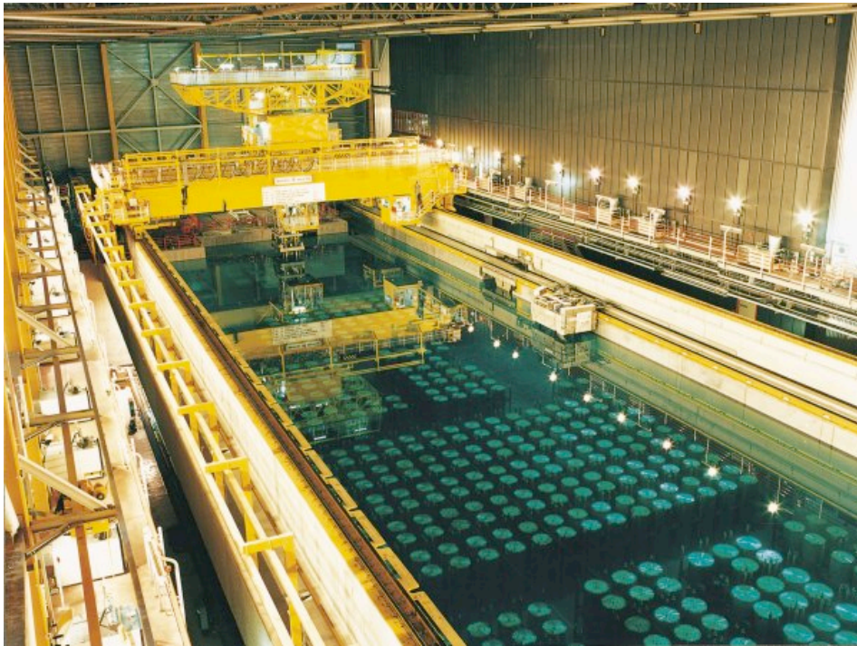
Storage pond for used fuel at the Thermal Oxide Reprocessing Plant at the UK's Sellafield site (Sellafield Ltd)
